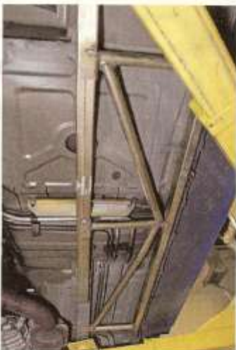
THE FINISHED product offers much more rigidity than the factory bolt-in connectors.
